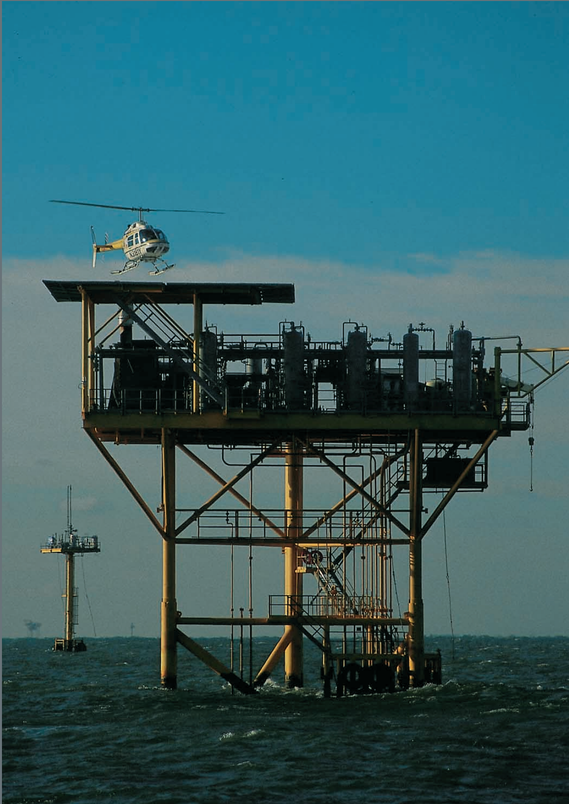
Production platform at South Pelto 1.
