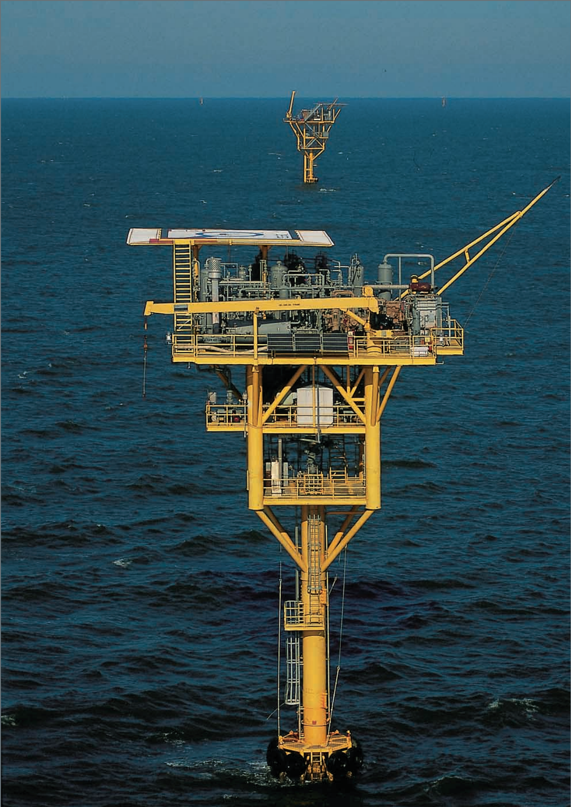
Ship Shoal 67 A production platform with Ship Shoal 66 B production platform in the background.
