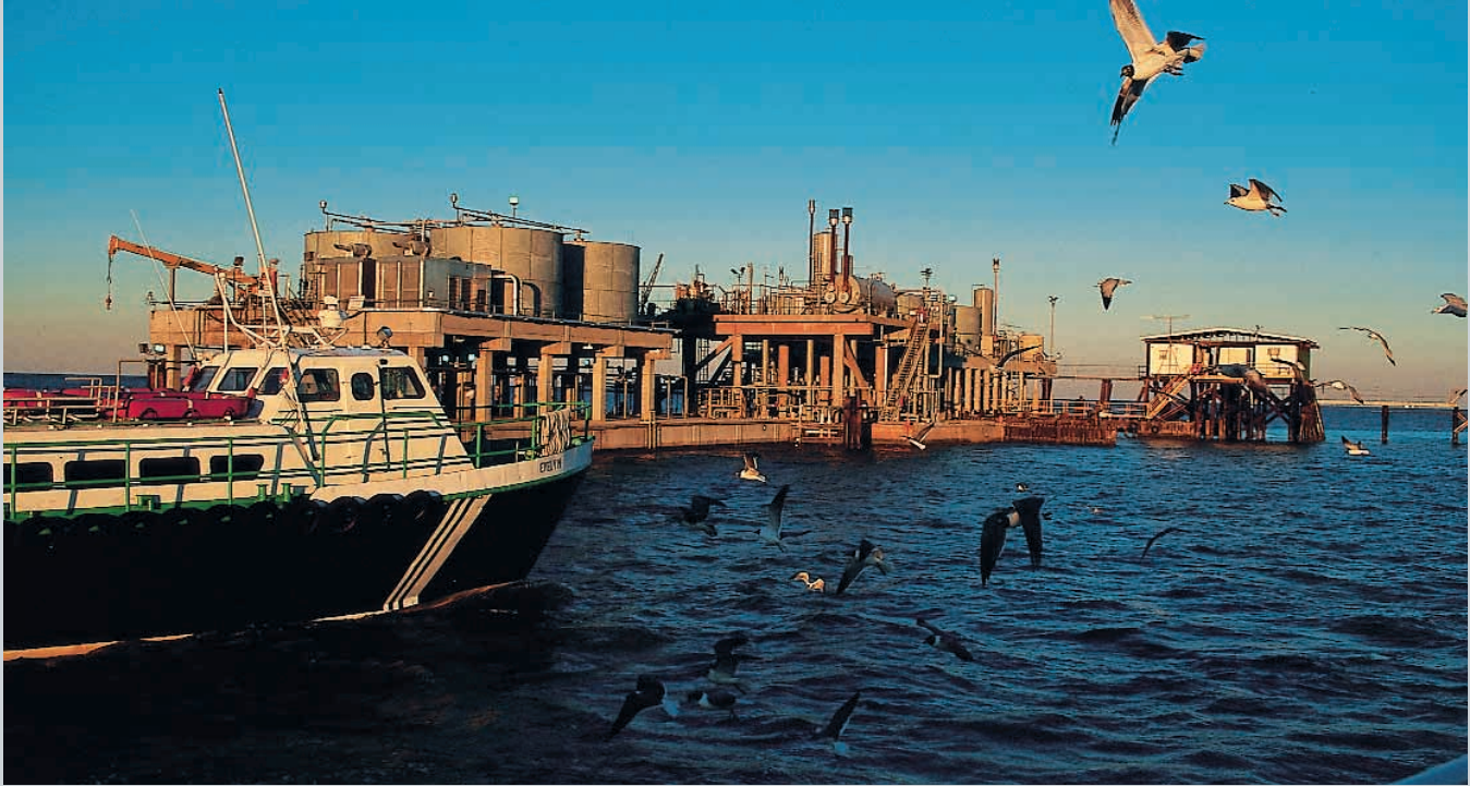
Central production and storage facility at Ship Shoal/South Pelto area.
